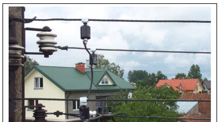
Fig. 4 ETITEC A limiters with clamp B for insulating line
