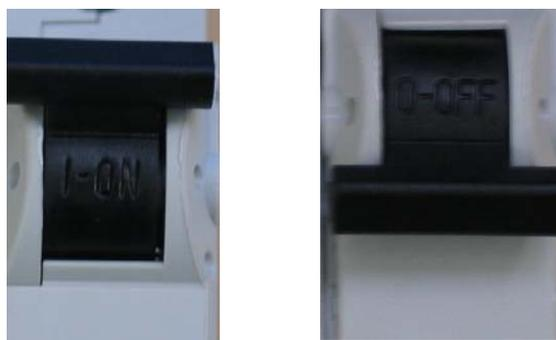
*Figure 2: ON-OFF button with indication "O – I" added on the circuit breaker*
